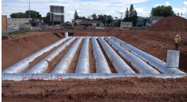
Subsurface Infiltration/ Detention
